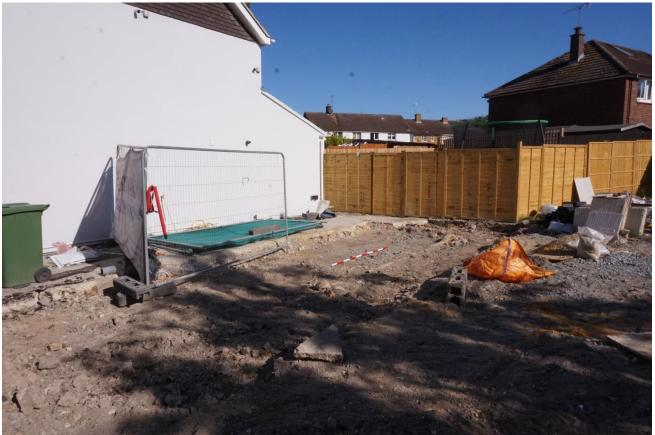
Plate 1: Looking north west at the site prior to trench excavation. Concrete floor and bedding was removed to the depth of 0.35m
